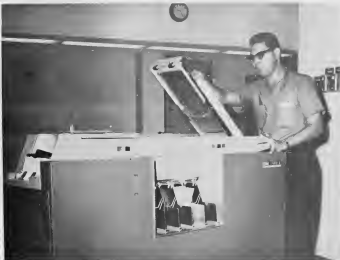
DATA CAN be read into the IBM 1492 reader-punch machine at the rate of 800 IBM cards a minute. Simultaneously, the unit can punch cards at the rate of 250 cards a minute with virtually no interruption of computing.
